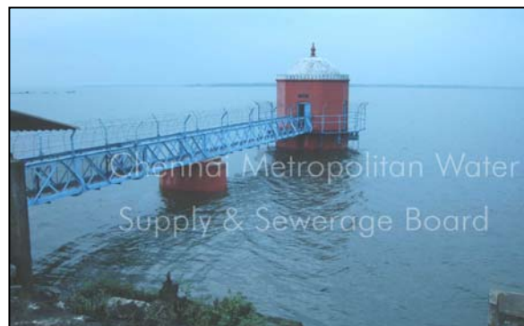
View of Redhills Reservoir
